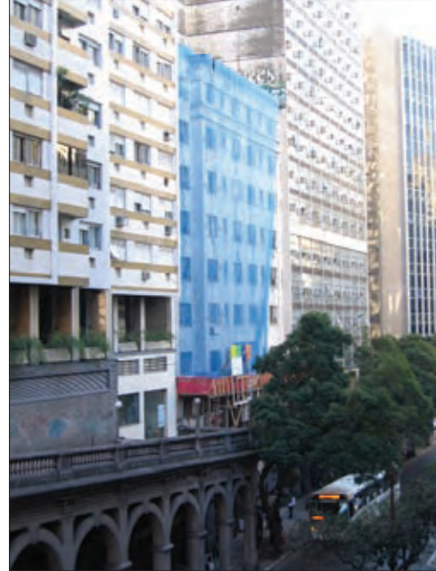
Picture 6: 14 July 2008, the building is being renovated.
