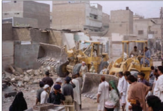
Picture 3: The demolitions.
