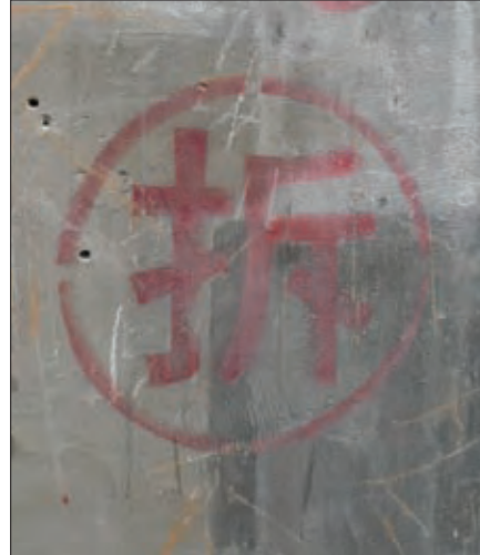
Picture 6: the dreaded symbol of a demolition order stamped on a building.
