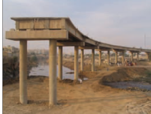
Picture 4: The construction of the LEW is underway.
